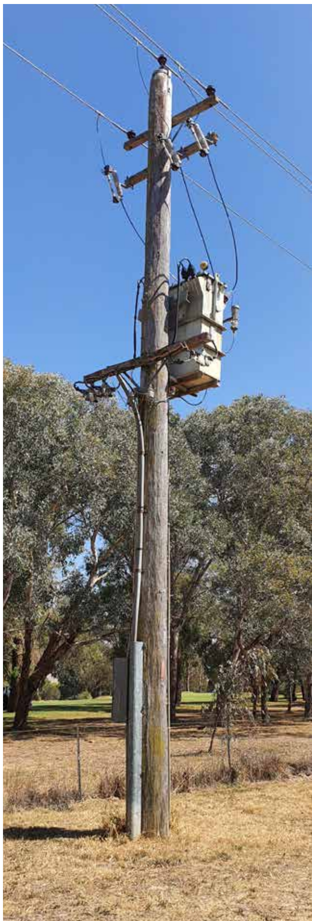
EVOENERGY DISTRIBUTION TRANSFORMER
