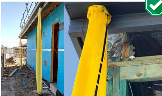
TEMPORARY DOWNPIPE EXAMPLES
