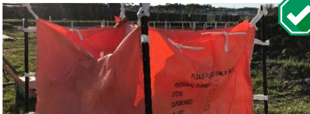
EXAMPLE OF WELL MANAGED WASTE/RECYCLING BAG
