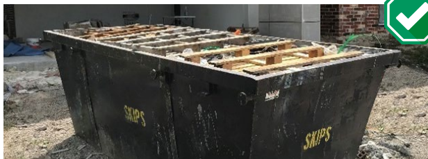
EXAMPLE OF WELL MANAGED SKIP BIN
