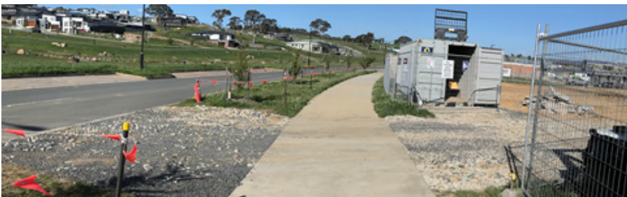
IMAGE 6: STABILISED ACCESS POINT
