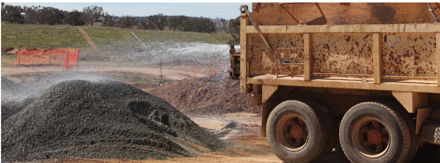
IMAGE 3: DUST CONTROL MEASURES
