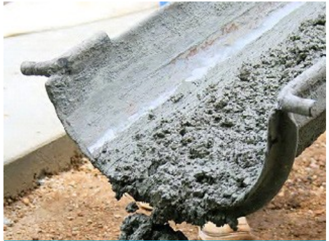
Chutes, barrels, wheelbarrows and other equipment must be rinsed in the site wash-down area.
